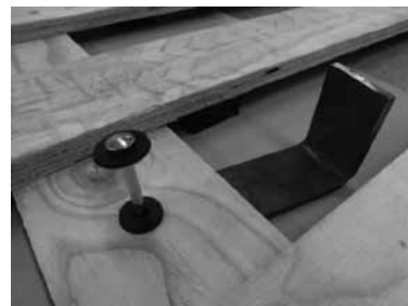
Hammer the anchor pin into place.
